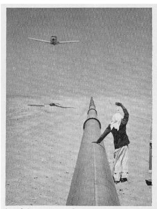
Low-flying company planes make weekly flights to inspect the pipeline that carries oil to the Mediterranean. Arabian American Oil Company.
